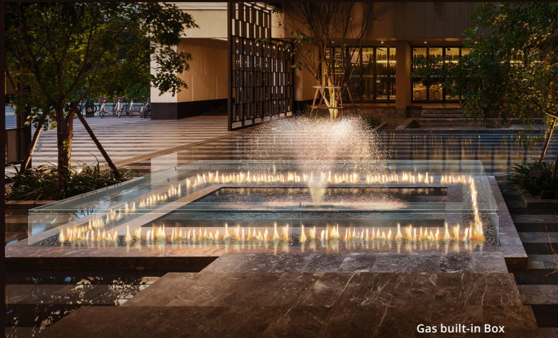
Gas built-in Box
